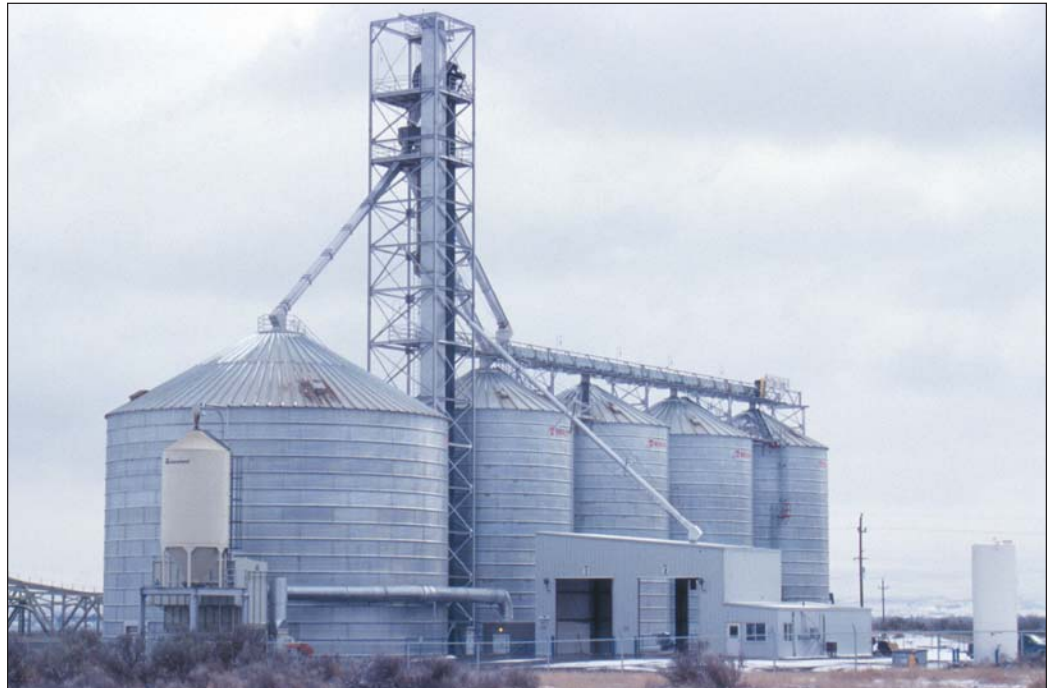
Tri-Cities Grain LLC's barge-loading terminal on the Snake River near Pasco, WA, features roughly 500,000 bushels of upright steel storage and another 2 million bushels in temporary storage capacity. Photos by Ed Zdrojewski.
