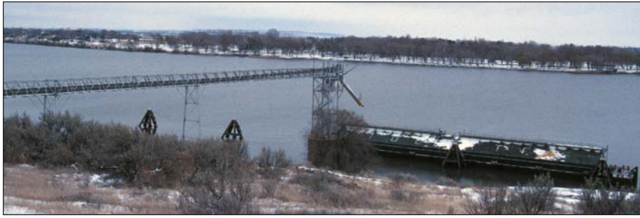
A 40,000-bph Hi Roller enclosed belt conveyor carries grain out to a computer-operated loadout spout for loading onto barges.
