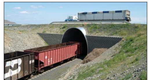
Portion of a 7,400-foot loop track runs through a 40-foot-deep culvert beneath the facility's truck entrance road.
